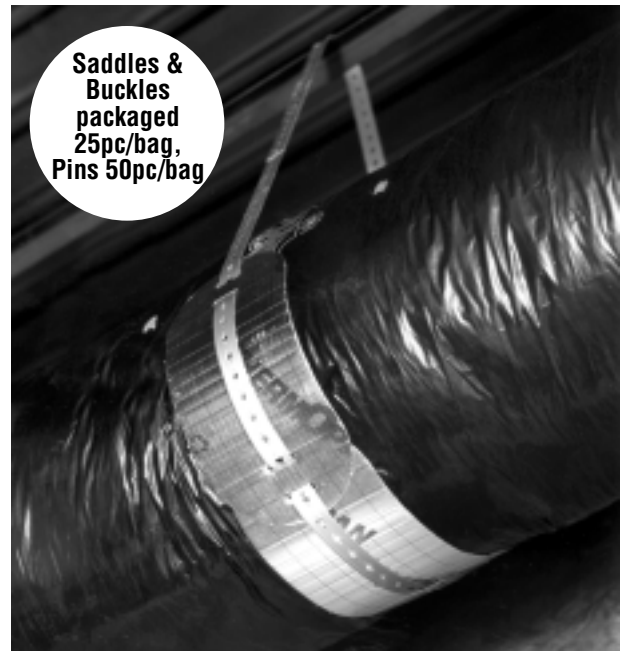
Link saddles together for larger duct application.
