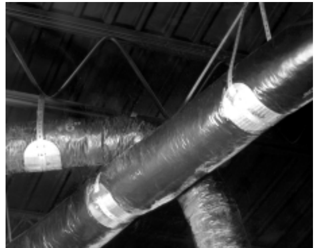
Use Saddles, Buckles and Pins with Thermo Button-Lok™, for a complete installation system.
