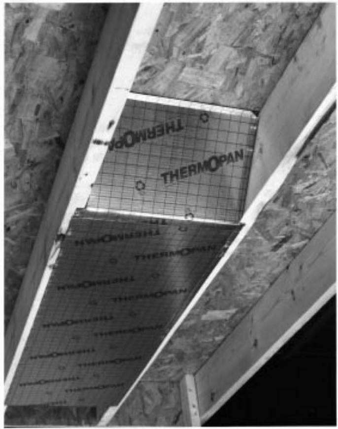
FIGURE 1—INSTALLED THERMO-PAN® PANELS
